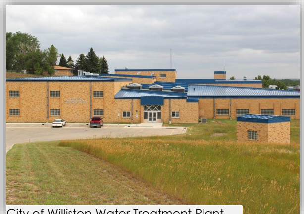
City of Williston Water Treatment Plant
